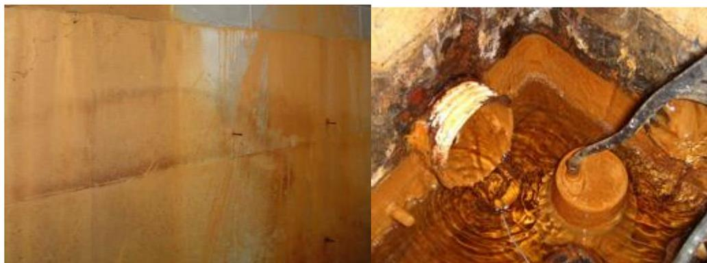
3. **Mold or mildew** – Dark stains on your wall are an indication of mold and/or mildew. These fungi are living, breathing organisms that grow in conditions where air, moisture and food are present. Mold and mildew can grow on or in walls (block or drywall), in carpeting, on furniture or anywhere else
